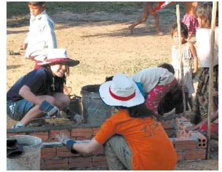
Laying the foundations for more greenery.
